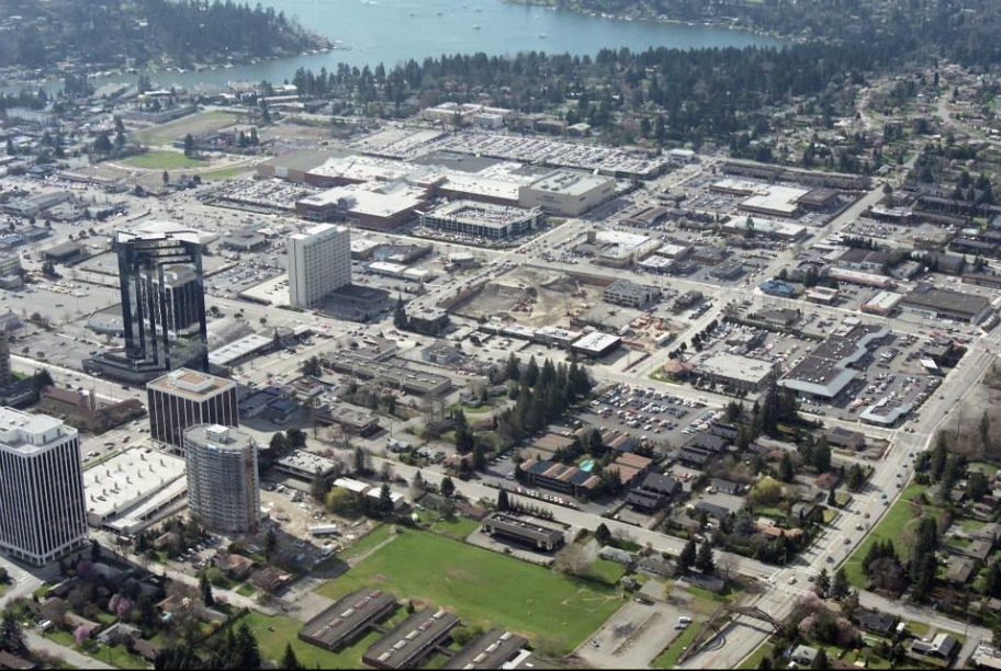
Bellevue Place/Bellevue Hyatt under construction. Bellevue, WA March 1987. Facing Meydenbauer Bay.
